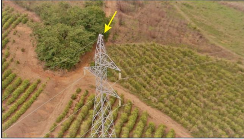
Figure 2 - Position of the lightning arrester on the right of Tower 8.
