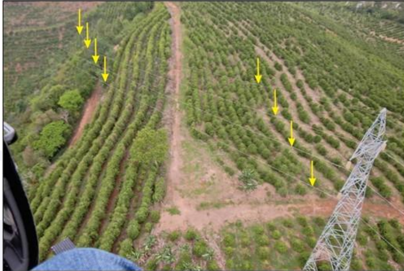
Figure 21 - Demonstration of the contrast of the cables and the tower, in relation to the terrain. The arrows indicate the positions of the cables between the two towers.
