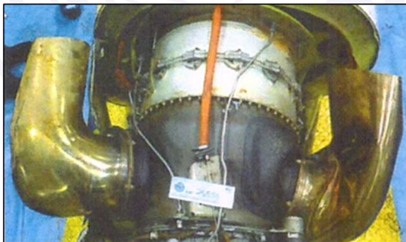
Figure 35 - Detail of the deformations of the lower part of the exhaust duct of the right-hand side engine.
