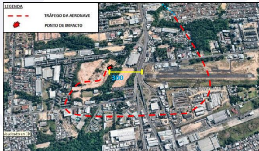
Figure 9 - Sketch of the accident showing the aerial view of the impact site and its position in relation to the threshold 11 of SWFN. The red dashed line represents the aircraft trajectory until the moment of impact.
