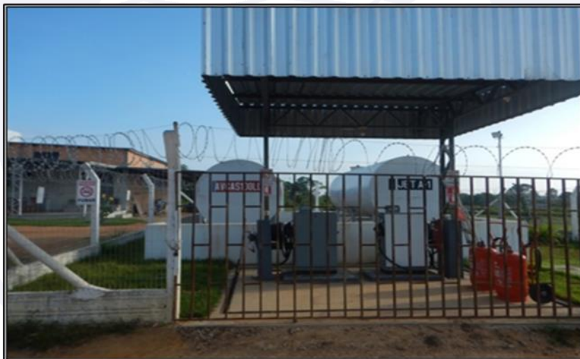
Figure 7 - Ethanol storage station of the company with the inscription of aviation kerosene (JET-A1).
