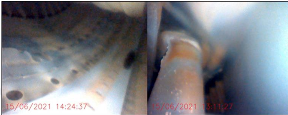
Figure 4 – Cracks in the combustion chamber and burn marks, erosion, and material loss in a compressor stator blade.
