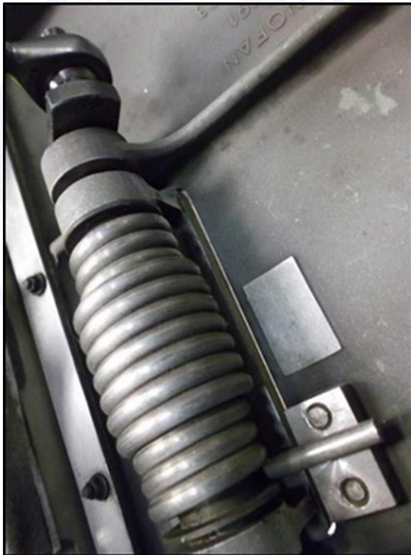
Figure 5 - Internal view of the small flap fully closed, after manual activation.
