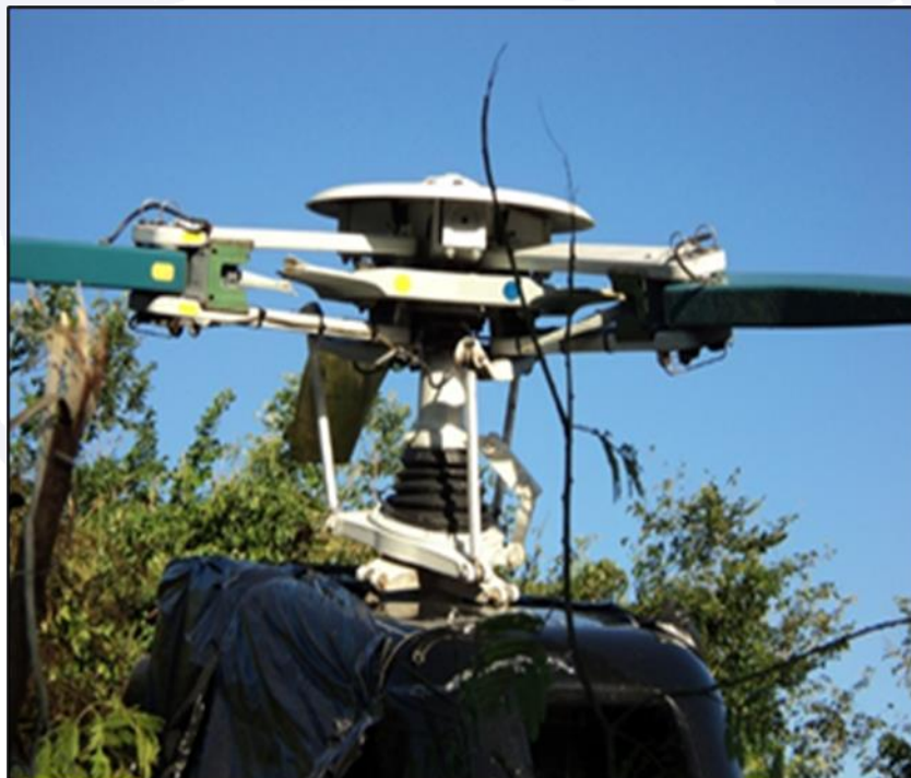
Figure 4 - Damage to the main rotor head.
