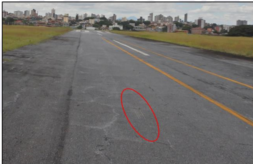
Figure 6 – Touchdown point of the aircraft, 180 meters short of the runway's end.
