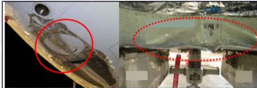
Figure 5 - Door frame location and deformation detail.
