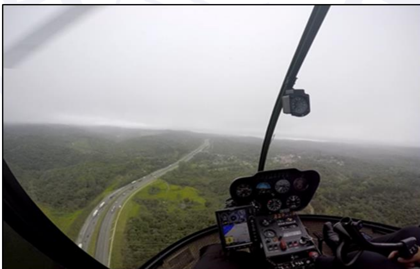
Figure 52 - 18:18:37 (UTC), overflight of a power grid network that passed on the BR-116, close to the bridge over the São Lourenço River.
