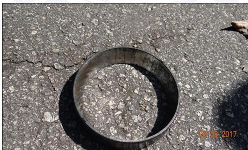
Figure 40 - Transmission case lower bearing outer race, undamaged.
