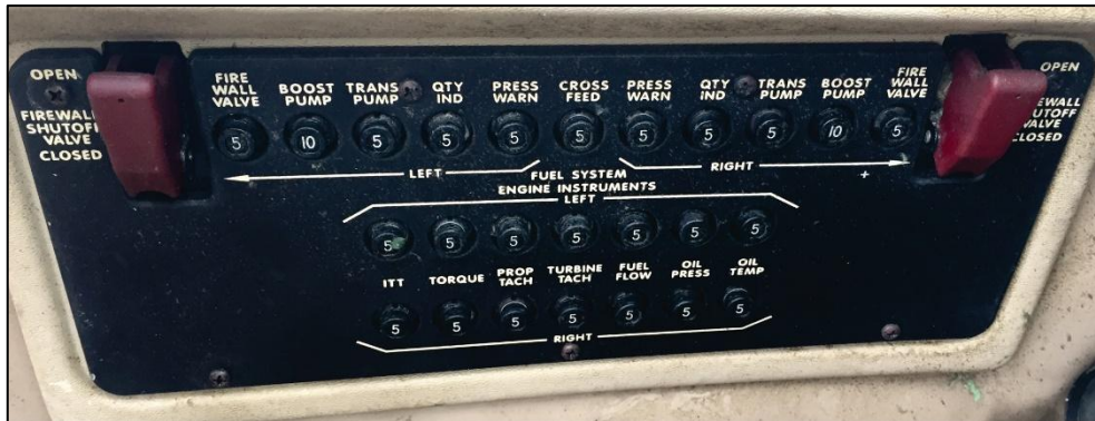
Figure 34 - Left circuit breaker panel.
