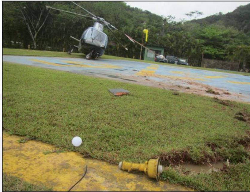
Figure 2 - Damage to the helipad beaconing.
