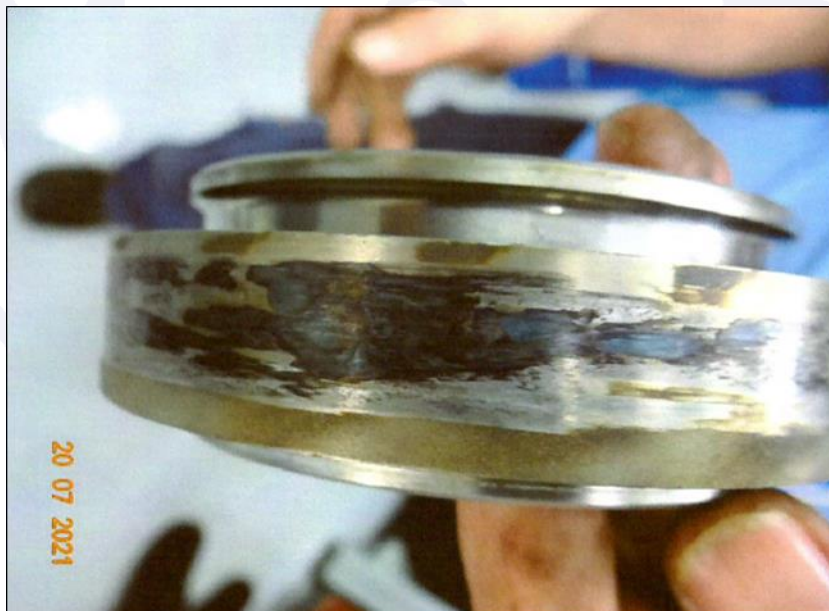
Figure 3 - Rubbing marks observed on the spacer between the 1st and 2nd compression stages.
