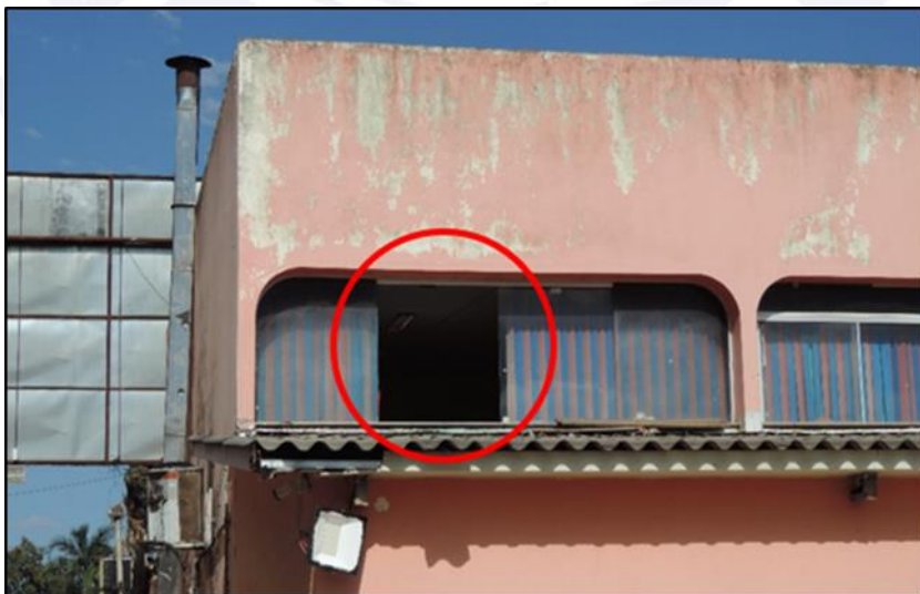
Figure 4 - Windowpane of a nearby building broken by debris.
