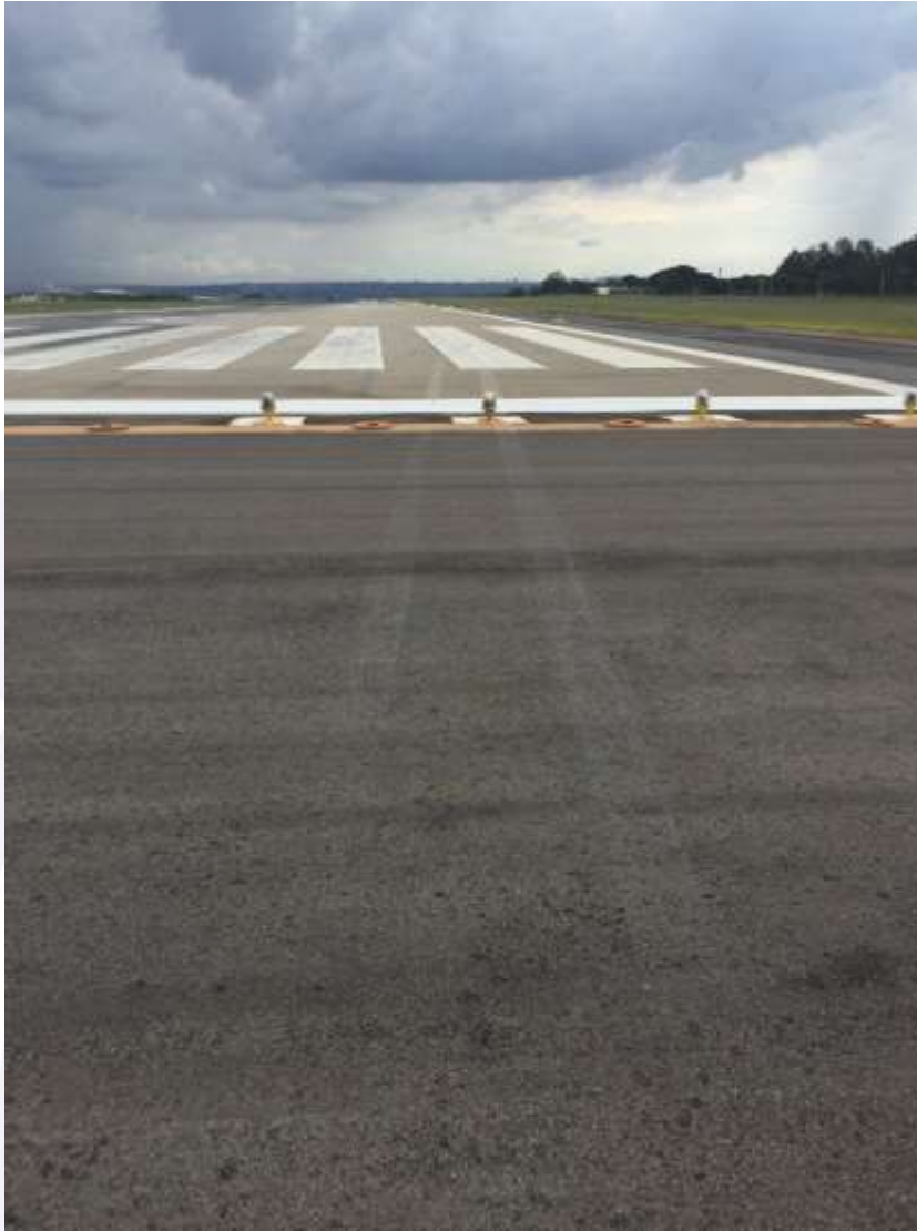
Figure 14 – Right main landing gear marks on RESA.
