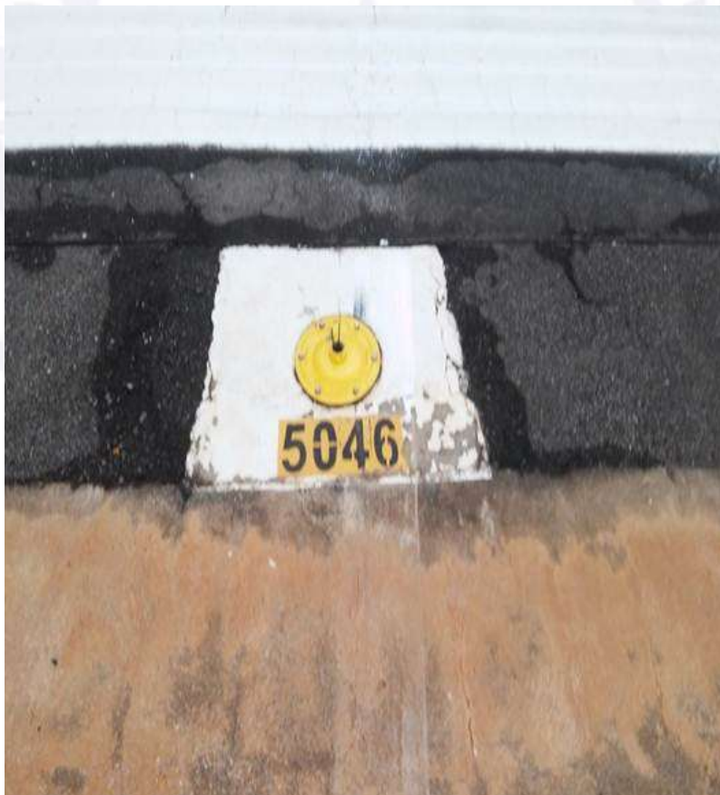
Figure 3 – Place where the struck threshold light was installed. (THR RWY29R)
