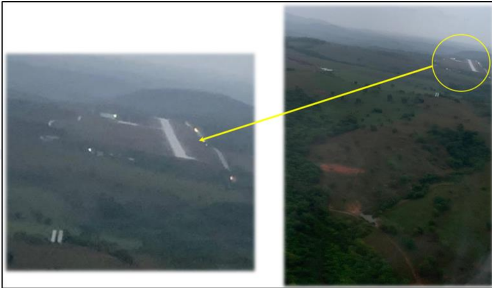
Figure 5 - Runway conditions on the day of the accident.
