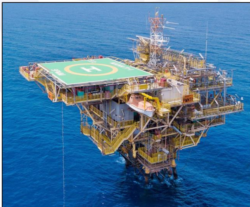
Figure 14 - Aerial view of the PMNT-1 Manati Platform (9PMM) helideck.
