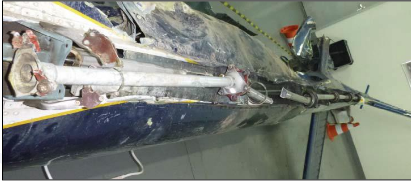
Figure 11 - General view of the tail rotor drive shaft assembly.
