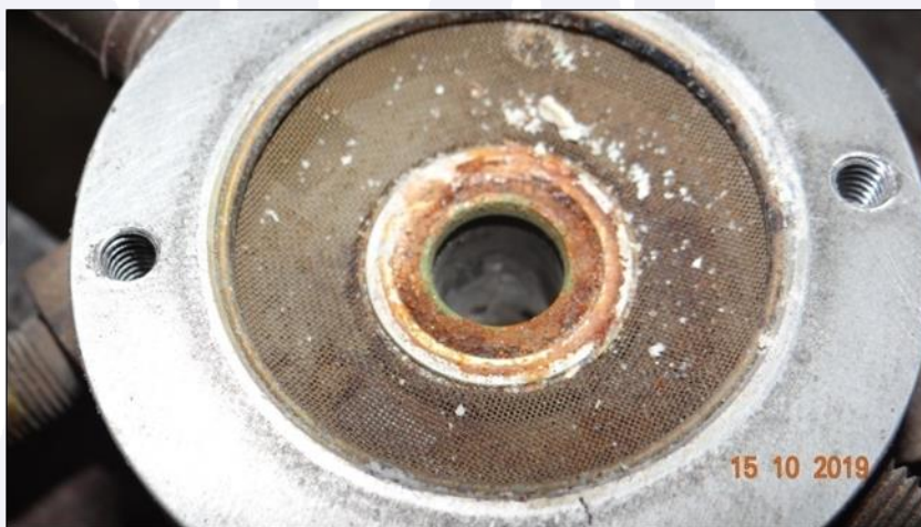
Figure 12 - View of corrosion in the distributor's internal fuel filter.
