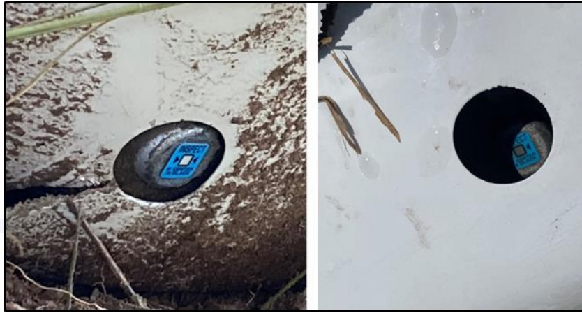
Figure 8 – Sequentially, the inspection windows for the left and right main gear.
