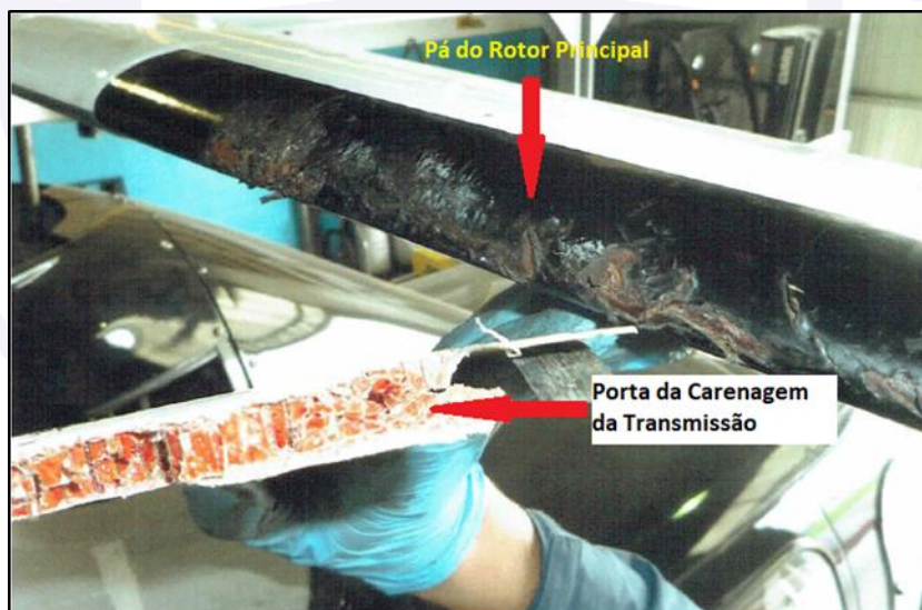
Figure 7 - Damage marks on the leading edge of the rotor blade and the fairing door.
