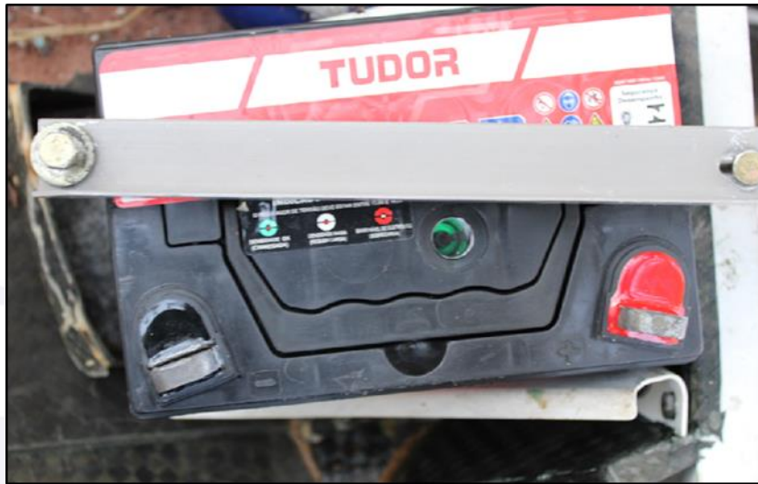
Figure 10 - Main battery installed on the aircraft.
