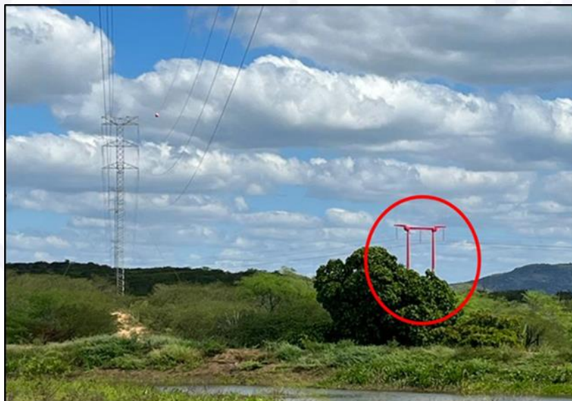
Figure 39 - Painting of 138-kV LT supports (towers), after the accident.
