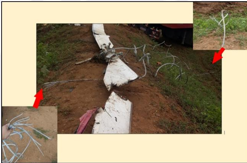
Figure 17 – Lightning-rod cable segment broken in two places (highlighted ends).
