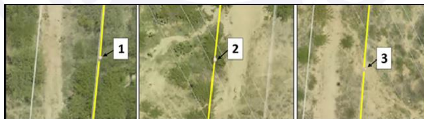
Figure 34 - Identification of the warning spheres of the electrical cables 1, 2, and 3, respectively, of the 230-kV LT.
