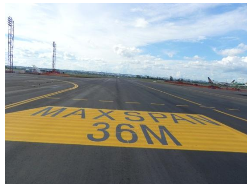
Figures 6 and 7 – Standard marking adopted by the ACI, and the marking on taxiway R, short of the entrance to taxiway L4.
