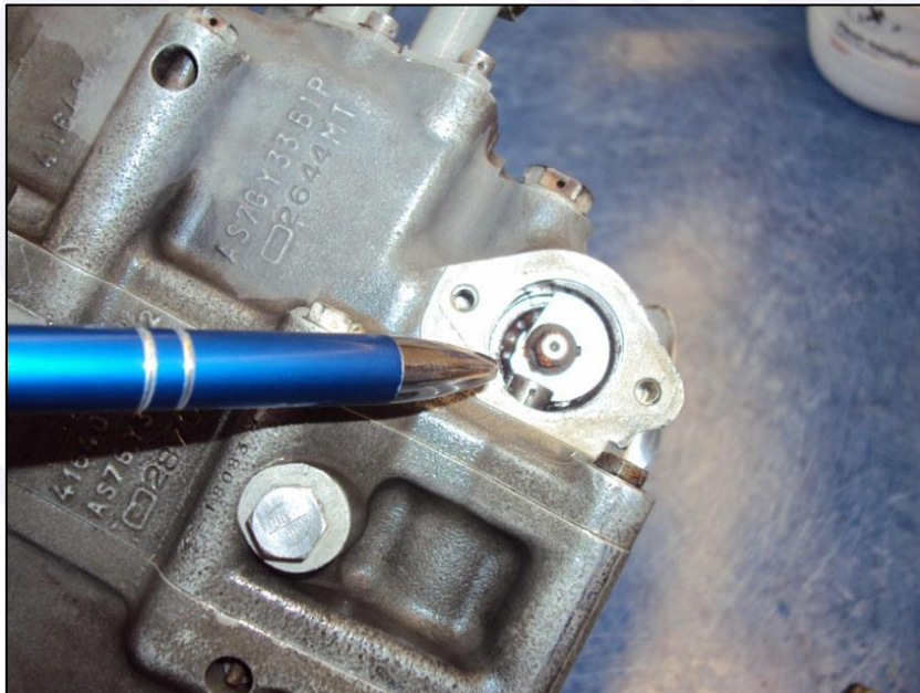
Figure 4 – View of the oxidation in the lid of the anticipator came before disassembly.
