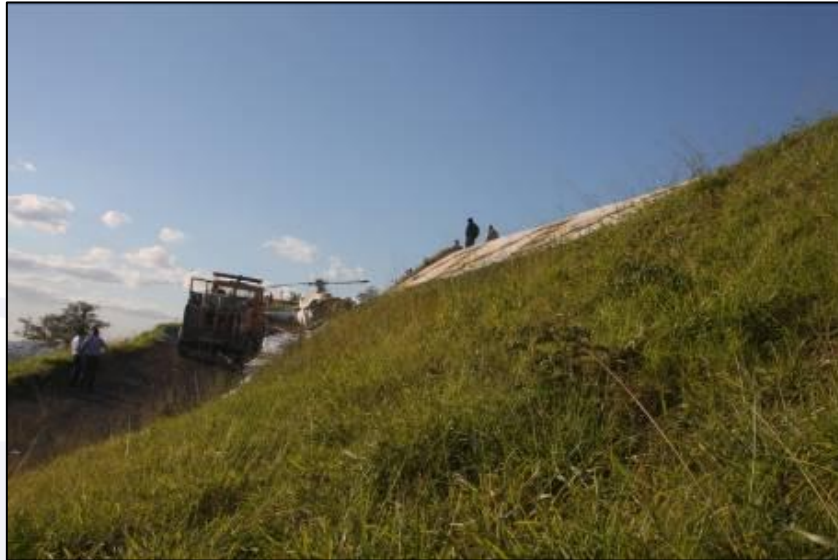
Figure 4 - Pronounced slope short of threshold 09.
