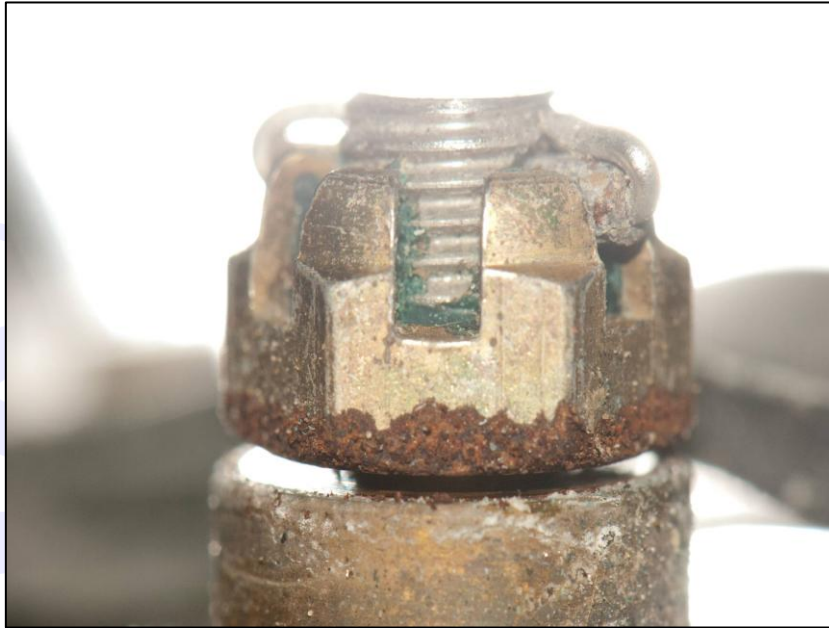
Figure 26 – Absence of corrosion inside the “stop” of the nut-bolt system.
