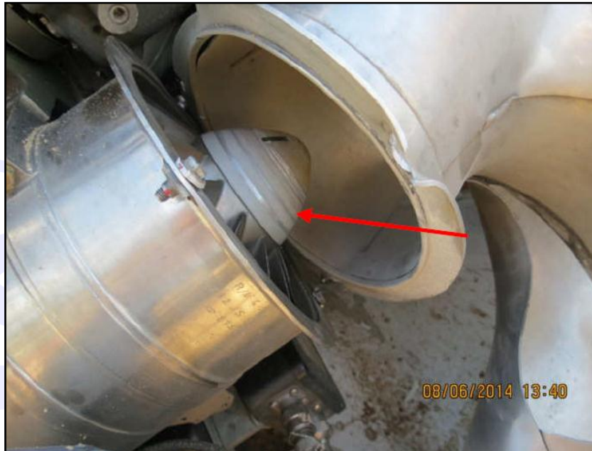
Figure 32 – Circumferential marks in the air inlet cone of the engine axial compressor.
