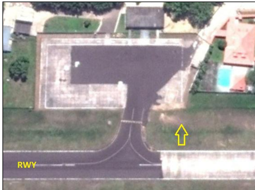
Figure 3 - Apron in relation to the runway (the arrow indicates the aircraft stop position)
