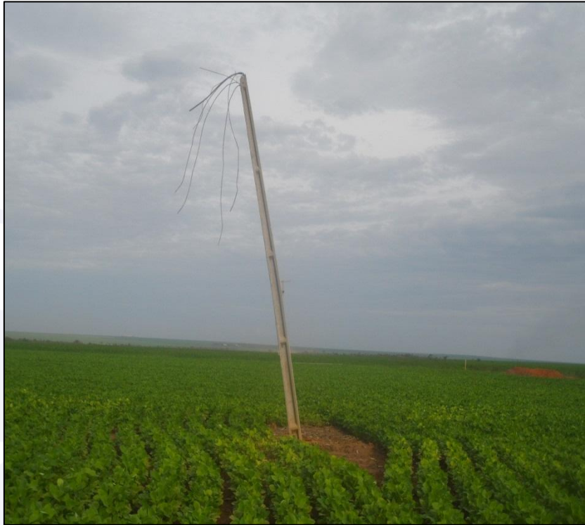
Figure 3 – Pole hit by the aircraft.
