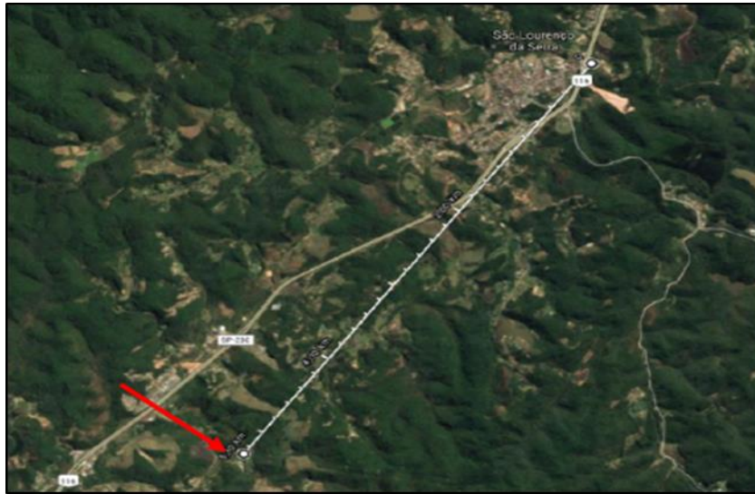
4 5 Figure 54 - Distance between the shed and the landing place, marked by the arrow.
