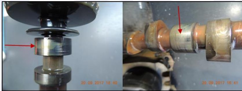
Figure 10 - Supporting bearings of the valve control shaft.
