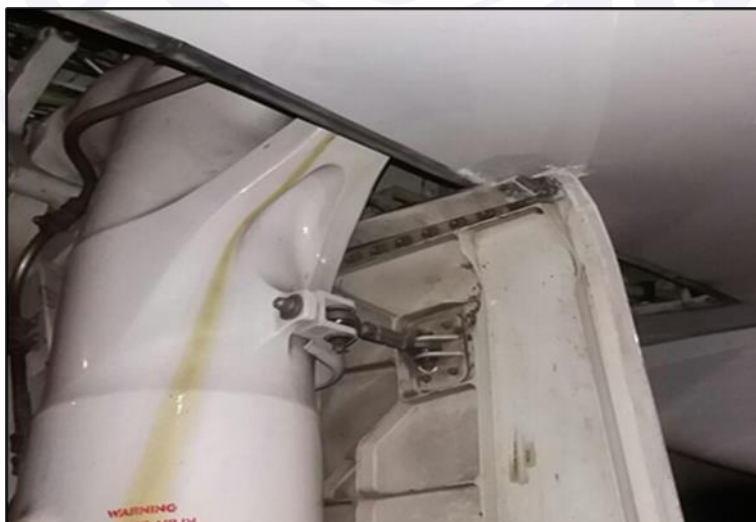
Figure 1 - Leakage of hydraulic fluid on the right landing gear.
