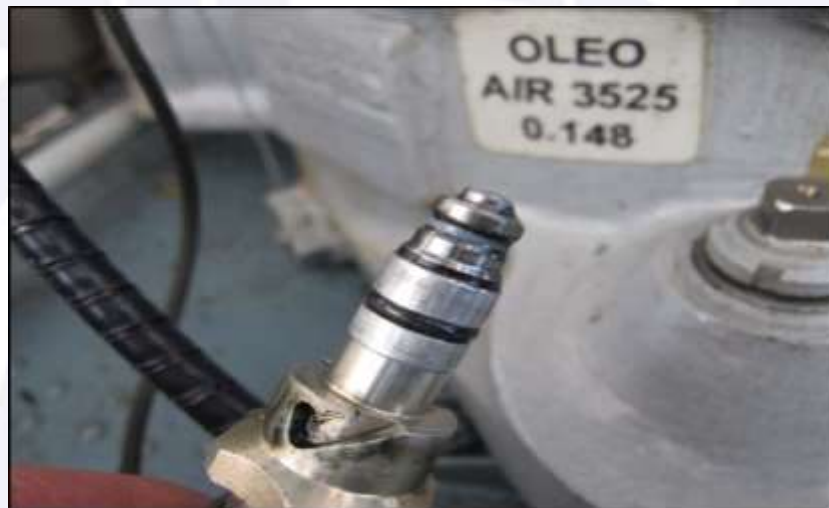
Figure 17 - Magnetic oil plug without particles or damage.
