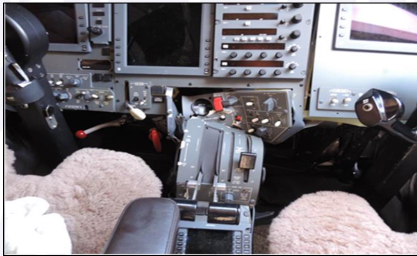
Figure 6 - Deformations in the aircraft panel and in the levers console. The right engine lever is already repositioned after the action of the fire brigade.
